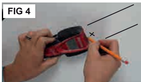
Mark Both Sides and Center of the Ceiling Joist
